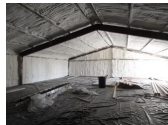
Insulation was done early 2017
