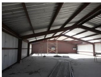
Roofing done in 2015-2016
